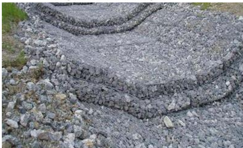
Figure 11-1: Example of Gabion and Reno structures
